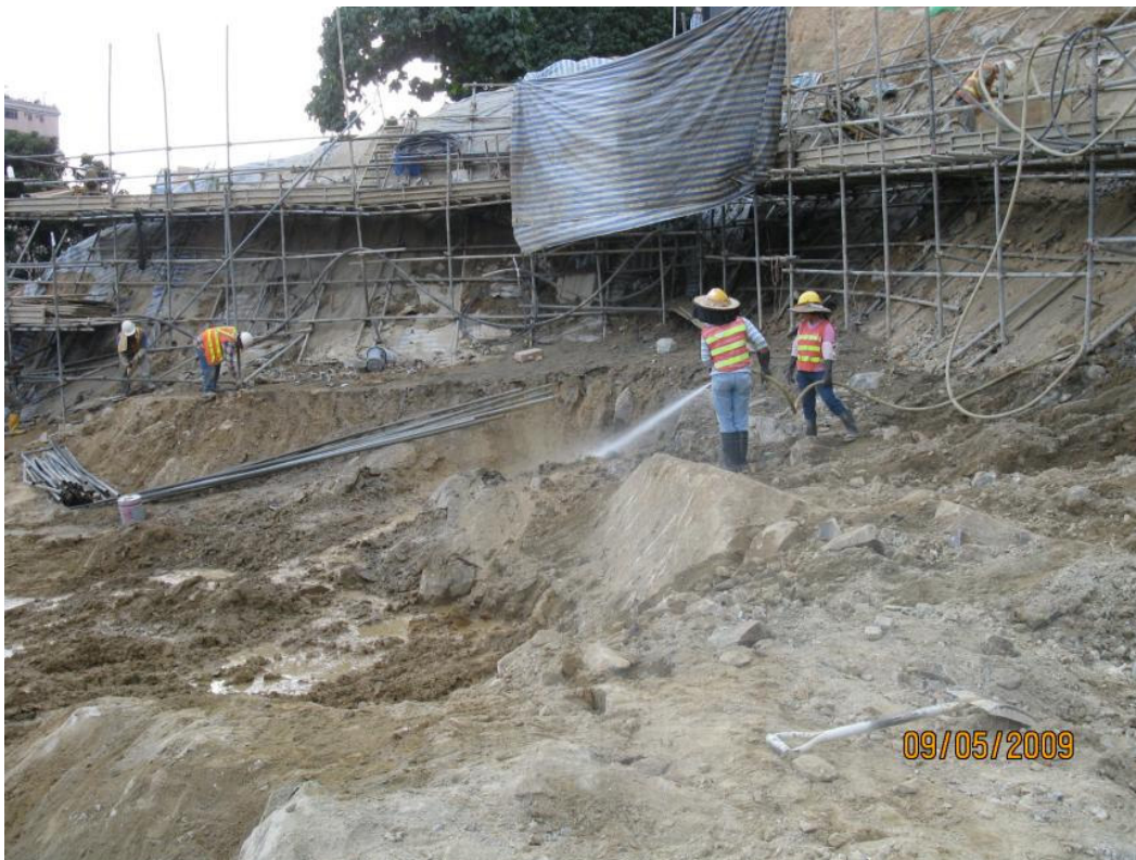
1. Water spraying for the exposed area.
