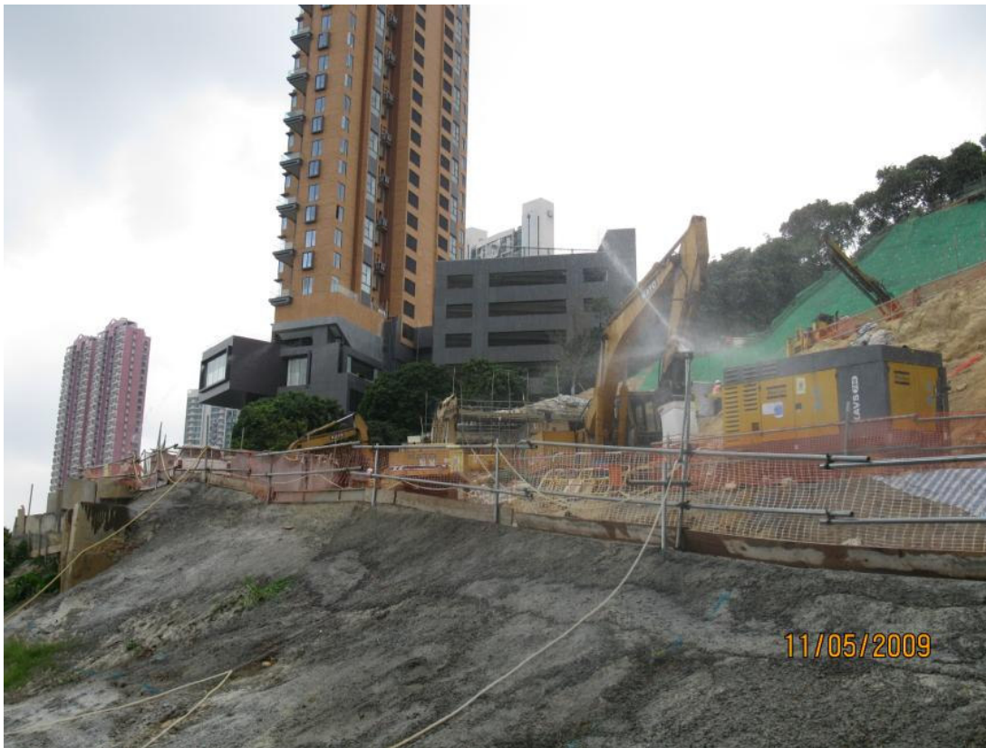
2. Automatic sprinkler spraying the haul road.
