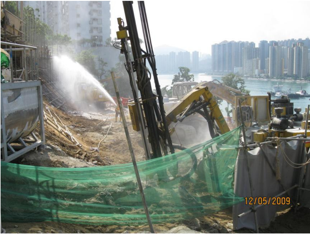
4. Water Spraying for soil nail work.
