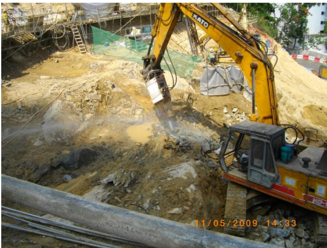
3. Water spraying during rock breaking.
