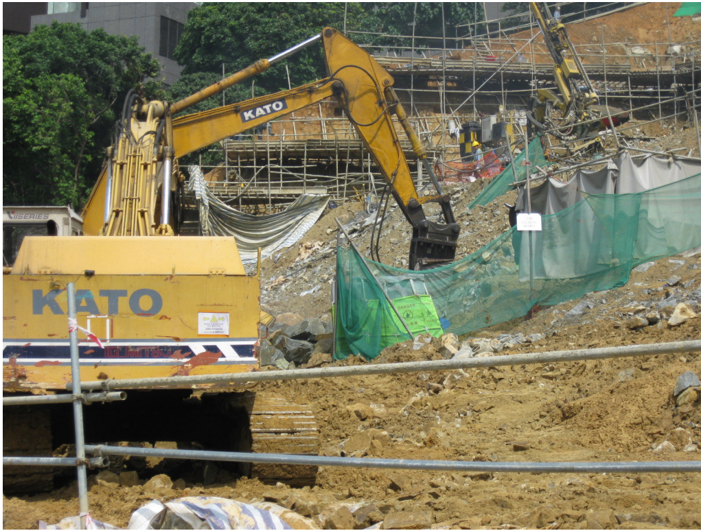
3. Noise insulation material for rock breaking.
